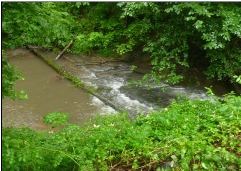
Photo 11 - Exposed 8-inch Distribution System Pipe in Elk Run
