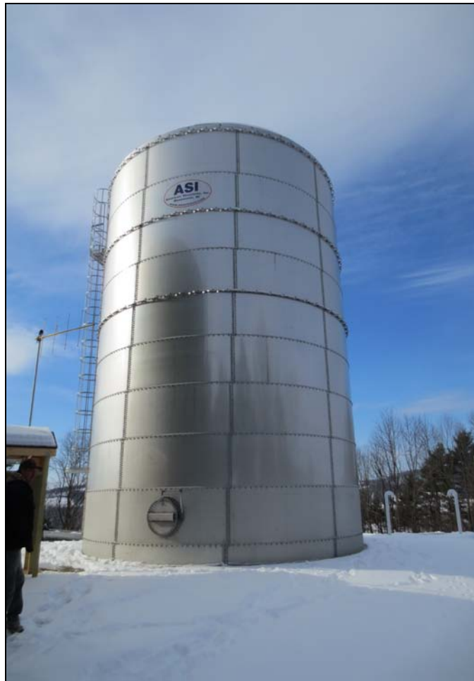
Photo 9 - Proposed Example of a Bolted Stainless Steel Ground Level Tank (165,000 Gallon Shown)
