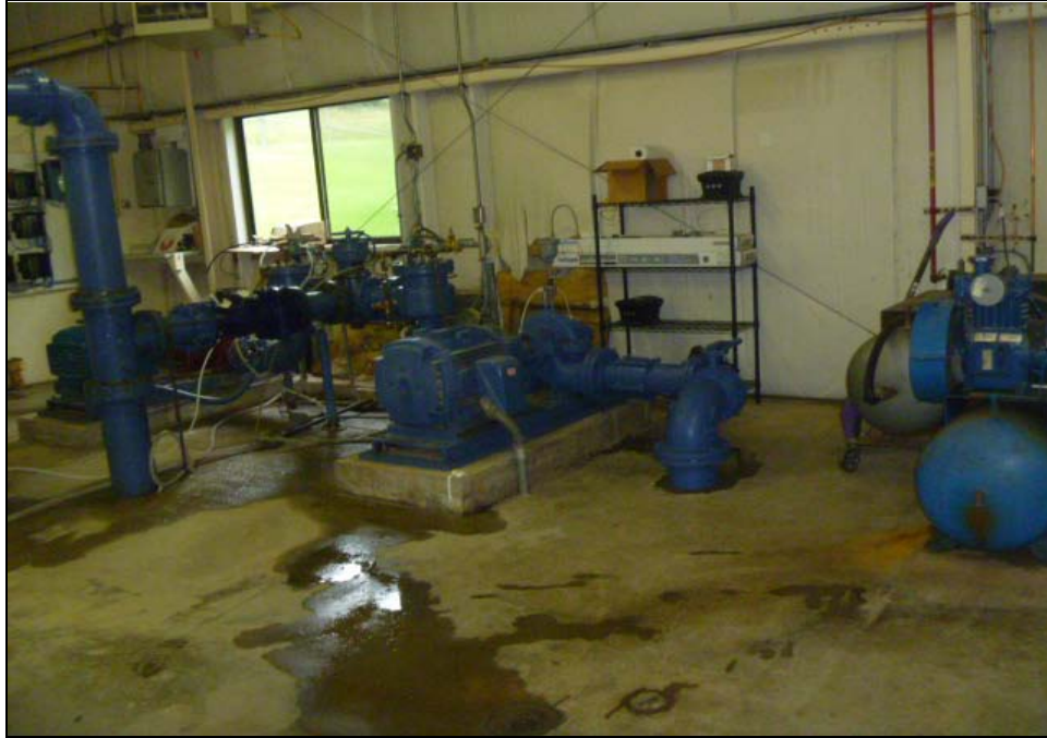
Photo 10 - Finish Water Pumps and Piping
