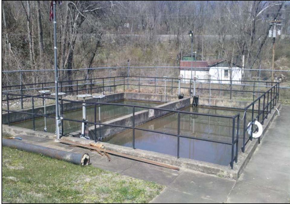
Photo 12 - Backwash Holding Tanks
