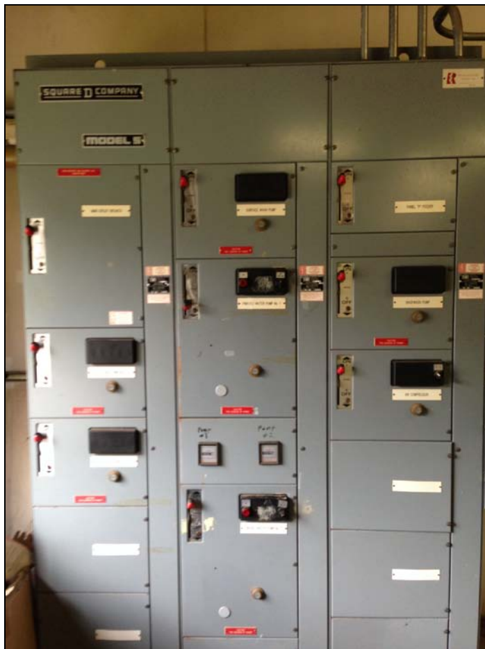
Photo 13 - Plant Motor Control Center
