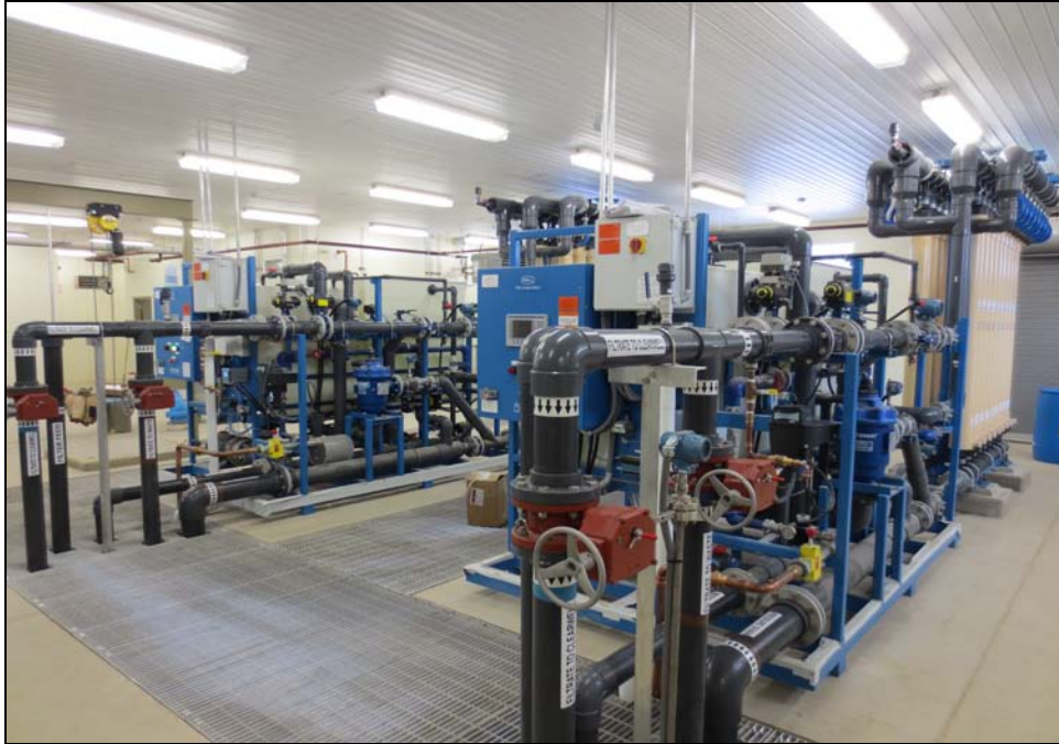
Photo 16 - Two (2) Proposed Membrane Skids (Pall Corporation AP-4s)
