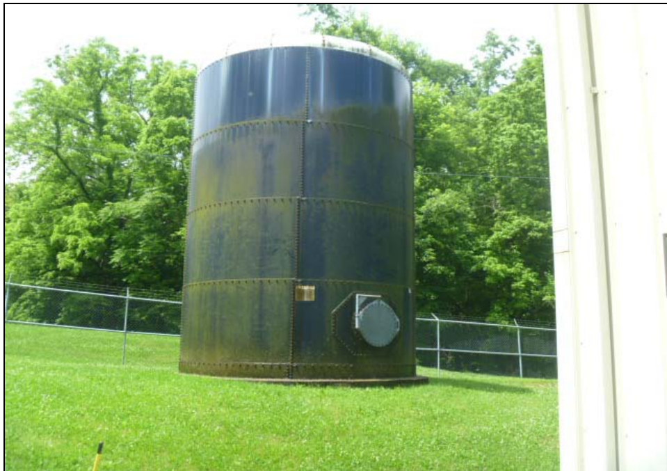
Photo 8 - Glass-Lined Ground Level Clearwell (21,000 Gallon)
