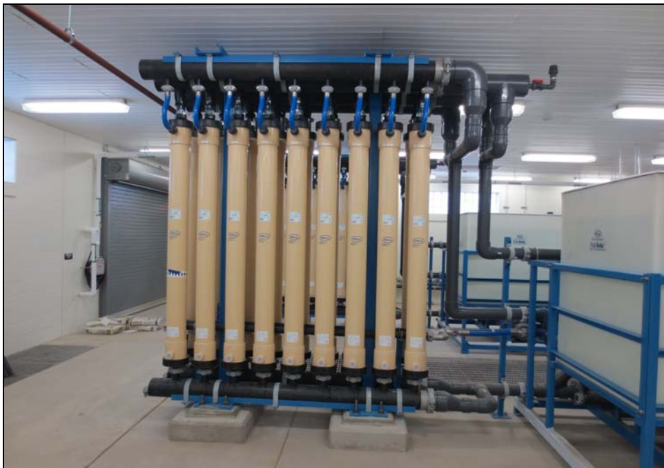
Photo 17 - Proposed Membrane Module Rack (18 Pall Corporation Modules Shown)
