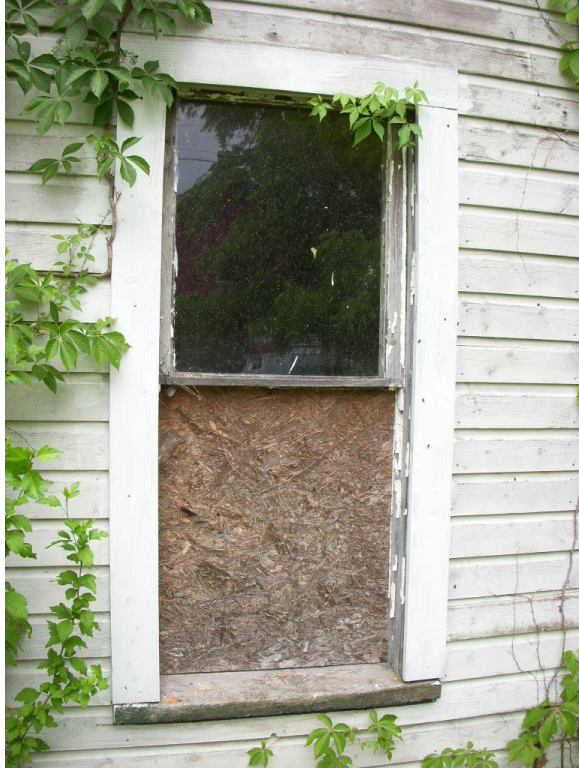
Existing window on west elevation of log building (west unit) with wood top sash having pegged connections (Oehrlein & Associates, 2008).
