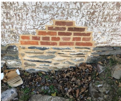
View of brick masonry repair (Mills Group 2018).
