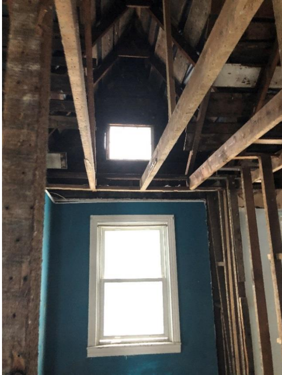
Central gable roof framing over second floor addition to log building, east unit (Mills Group, 2018).
