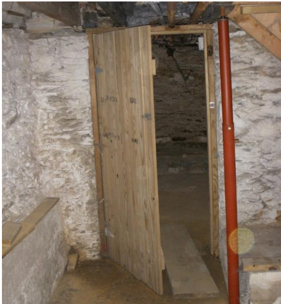
View to north from the cellar under the main portion of the building into the cellar under the rear wing showing original stone wall opening and modern door and frame construction (Oehrlein & Associates, 2008).
