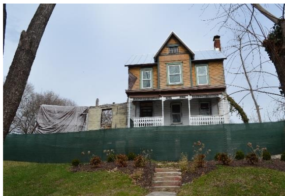
Photograph of south elevation of property illustrating deterioration of west half of duplex (Mills Group, 2018).
