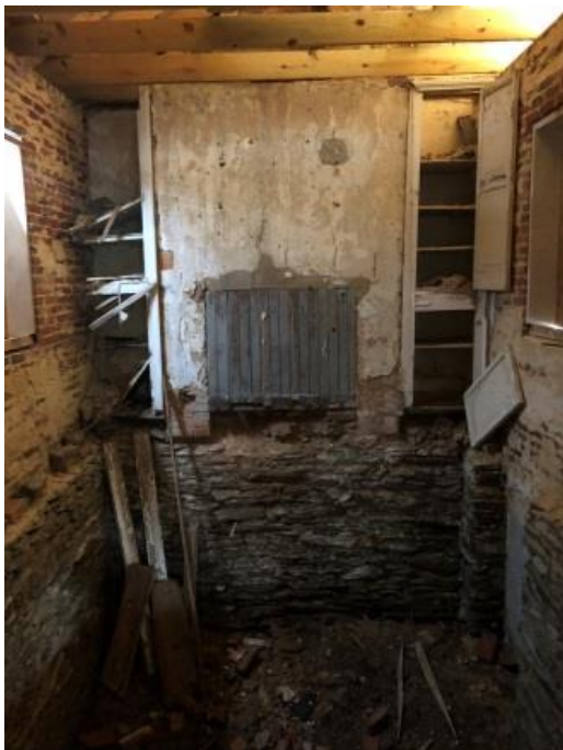
View of missing floor framing in rear wing (Mills Group 2018).
