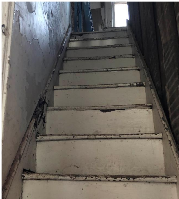
Wood stair assembly from first floor to second floor level (Mills Group 2018).
