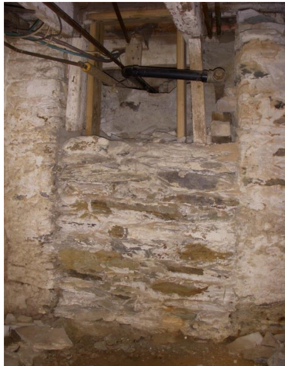
Original opening in east wall of cellar below rear wing, partially filled in with fieldstone. Note the existing floor joists above that are supported by two wood posts (Oehrlein & Associates, 2008).
