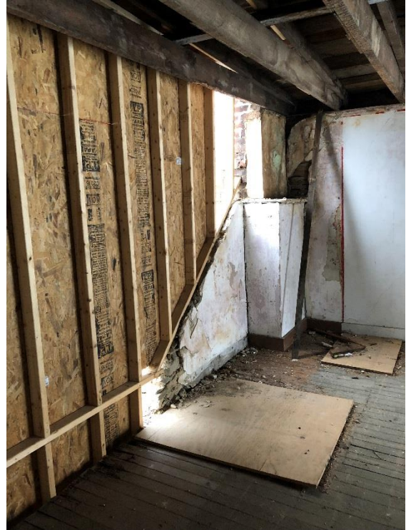
Frame wall on west side of east unit second-story addition to stone building (Mills Group, 2018).
