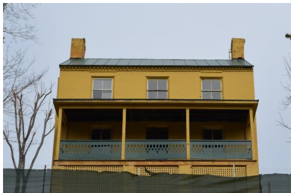
View of out-of-plumb chimneys on main building (Mills Group 2018).
