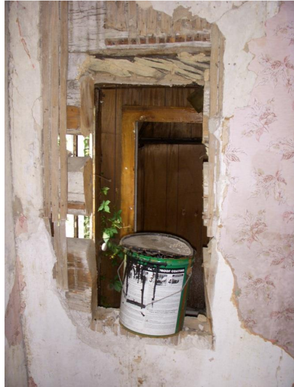
Opening made in north wall of west unit log building (Oehrlein & Associates, 2008).
