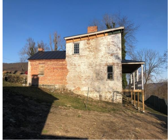
West elevation showing rebuilt rear wing walls (Mills Group 2018).
