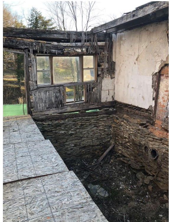
View of deteriorated picture window opening, West Unit log building (Mills Group, 2018).
