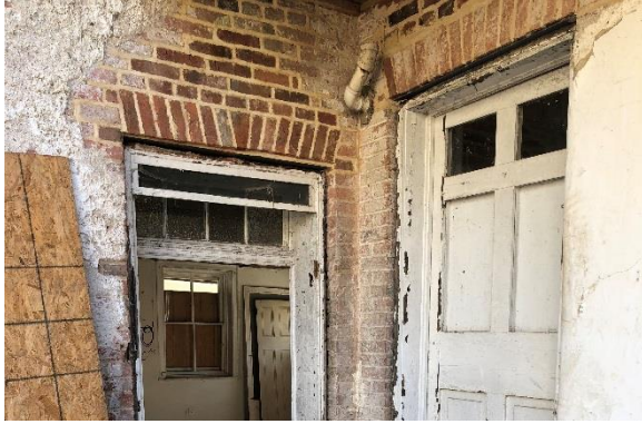
Reconstructed jack arch and adjacent masonry over exterior door opening on north wall (Mills Group 2018).
