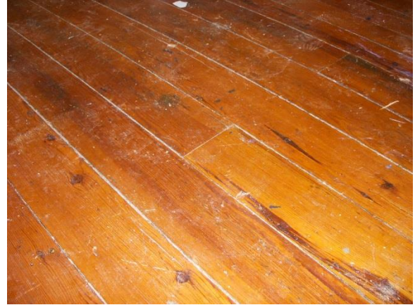
Interior floorboards of random length and width (Oehrlein & Associates, 2008).
