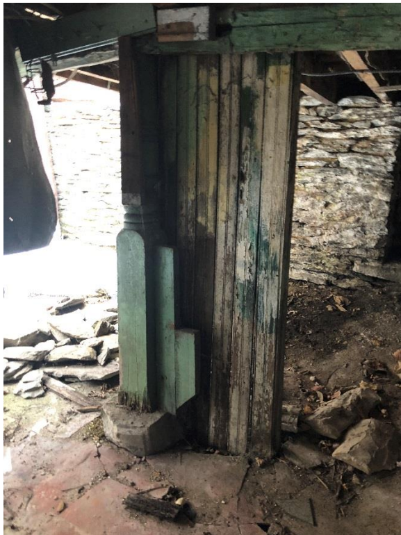
View of single post currently supporting West Unit floor framing (Mills Group 2018).
