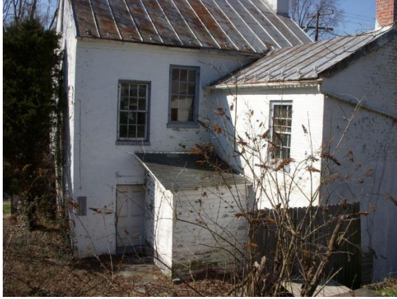
View of north elevation of main building and east elevation of rear wing. The wood-framed shed was added after 1933 (Oehrlein & Associates, 2008).
