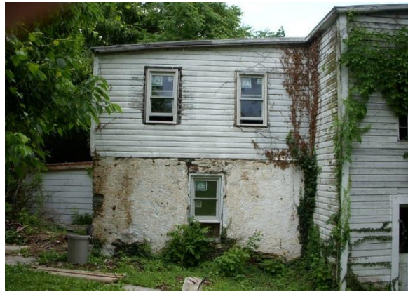
Shadows at the second floor windows of the west unit indicate the former presence of shutters at these windows (Oehrlein & Associates, 2008).
