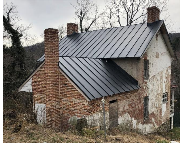
View of new sheet metal roofing and flashing (Mills Group 2018).
