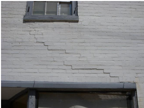
View of crack in masonry wall at south elevation (Oehrlein & Associates, 2008).
