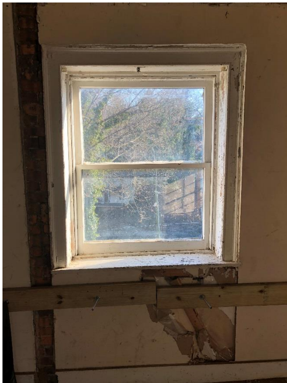
Non-original 1-over-1 double-hung wood windows (Mills Group 2018).
