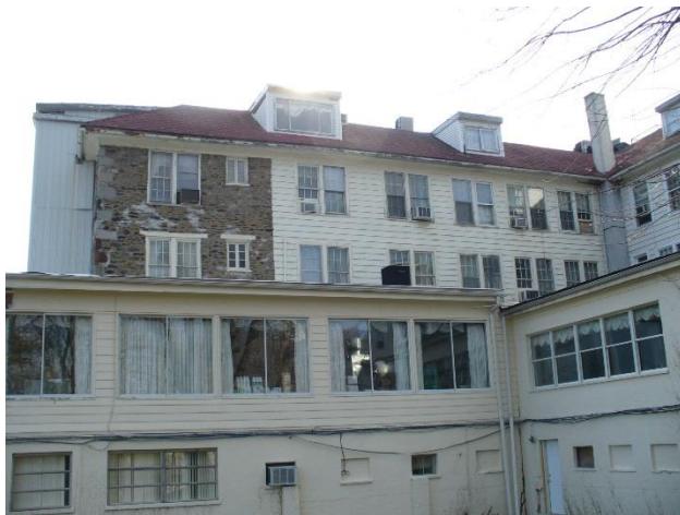
Area 1 west elevation showing the 1920 stone and frame wall construction, recent roof dormers and recent concrete block and frame additions. A portion of the stone wall may date from the 1913 reconstruction. The corner quoins appear similar to those in the 1914 west elevation photograph.
