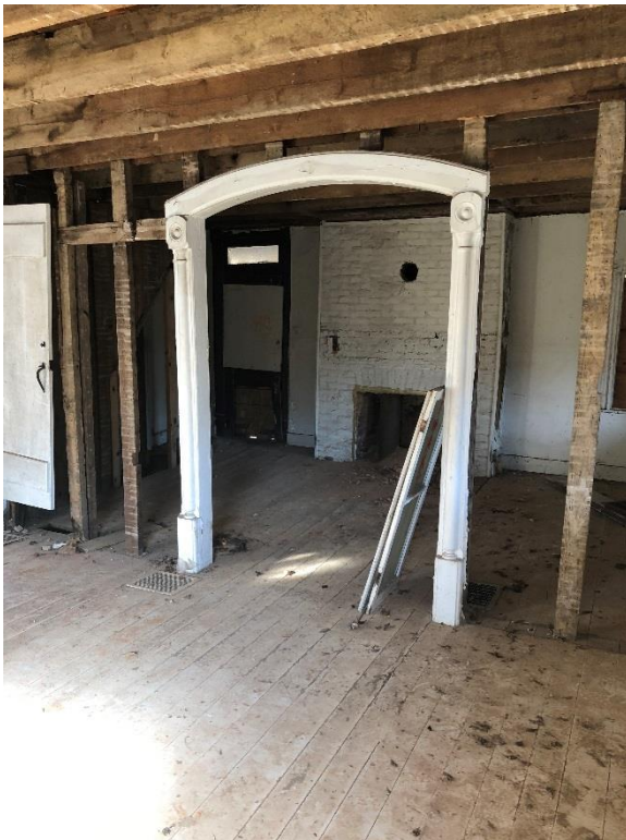
Existing interior door trim; clean, repair, prime and paint all elements scheduled to remain (Mills Group 2018).
