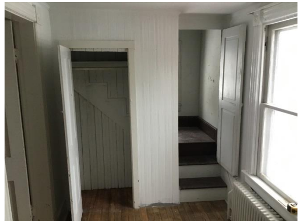
Attic stair entrance and adjacent closet showing stair carriage (Mills Group 2018).
