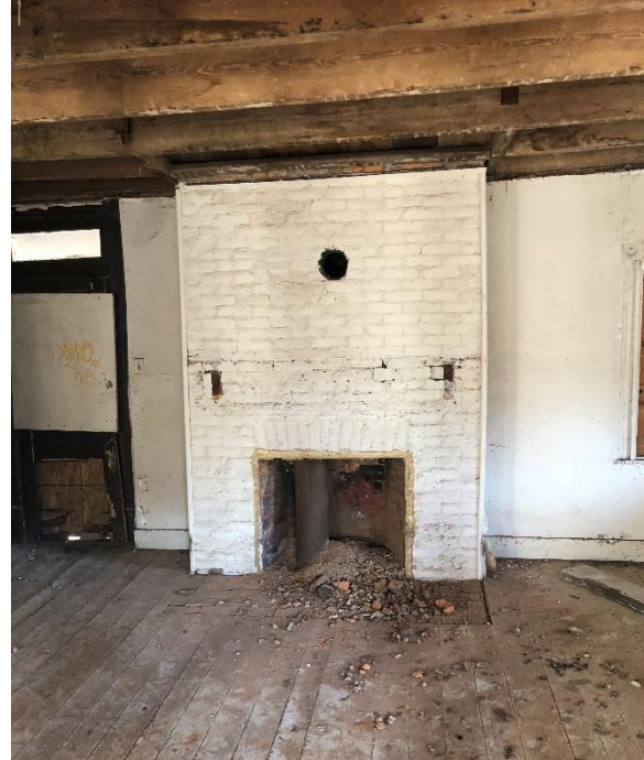
View of missing mantle at east fireplace on first floor; replicate west fireplace mantle for installation (Mills Group 2018).
