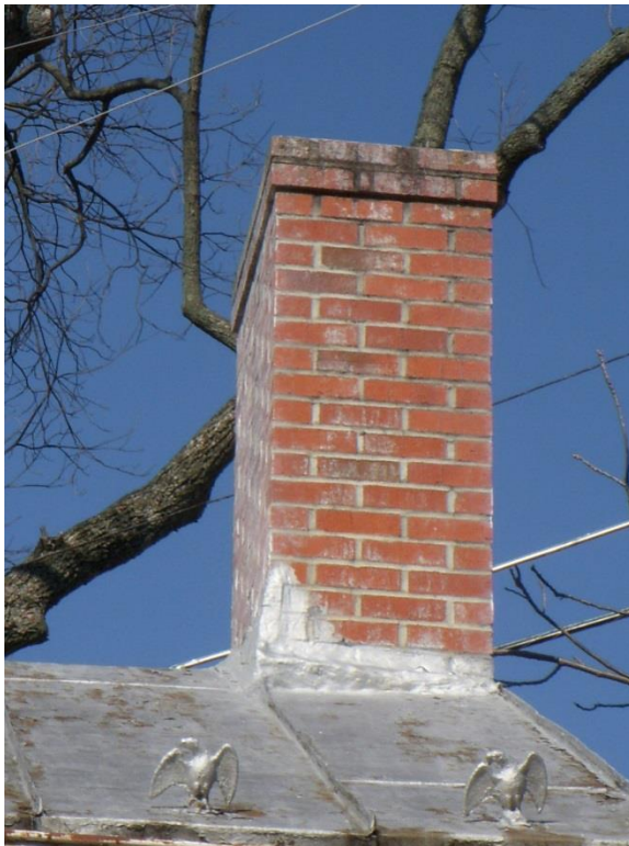
Chimney on rear wing that has been recently reconstructed. Note the decorative eagle snow guards (Oehrlein & Associates, 2008).
