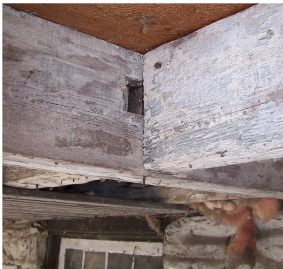
Mortise-and-tenon porch floor structure (Oehrlein & Associates, 2008).
