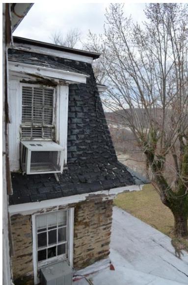
Asphalt shingle roofing (Mills Group, 2018).
