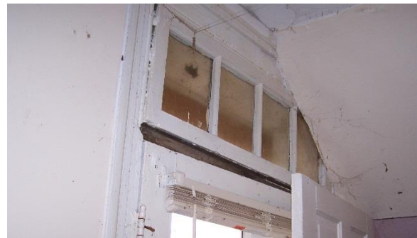
Detail stair bulkhead at transom over north entry (Oehrlein & Associates, 2008).
