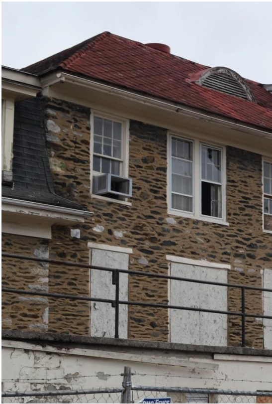
Wood windows and missing windows at stone and frame walls (Mills Group, 2018).
