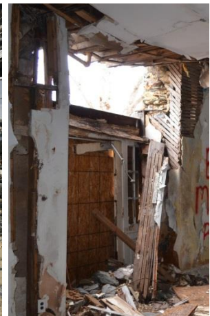
Interior view of deterioration of east wall (Mills Group, 2018).
