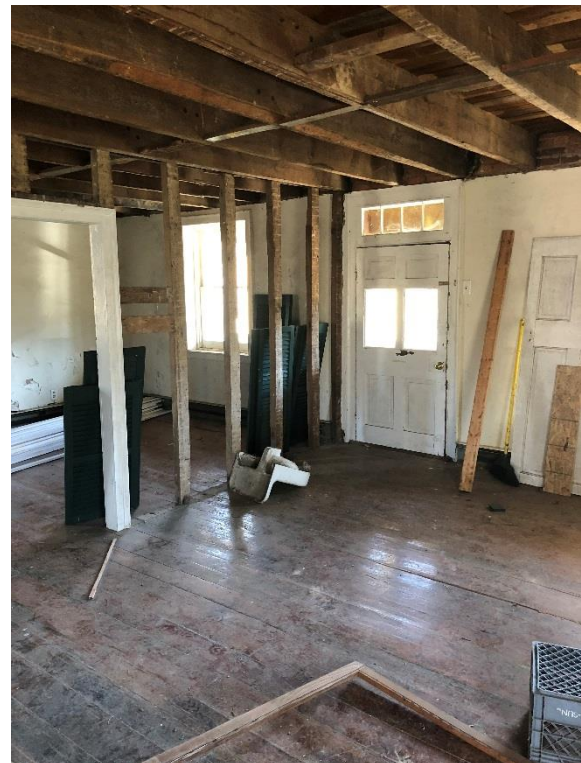
Interior framing with plaster and lath removed (Mills Group 2018).
