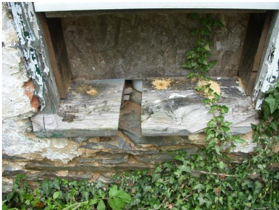
Existing window opening in west elevation of stone building (west unit). Brick masonry on the left side of this opening indicates that the width of the opening may have been modified over time. Also note the portion of wood removed from the wood sill (Oehrlein & Associates,
