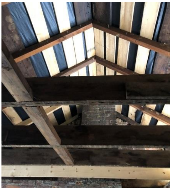
Rehabilitated roof framing over rear wing (Mills Group 2018).
