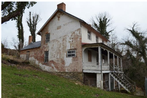
View of deteriorated stucco on west elevation (Mills Group 2018).
