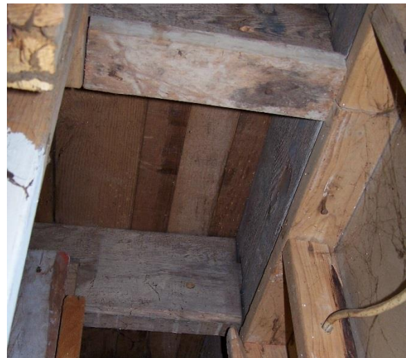
Framing of stair at first floor. Modern framing contrasts with original tenoned floor joists (Oehrlein & Associates, 2008).
