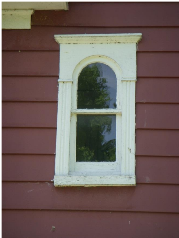
View of second floor window, east side of north elevation. This window is very similar in detail to the pair of windows in the cross gable of the south elevation, and may have been relocated when the rear wing was expanded (Oehrlein & Associates, 2008).
