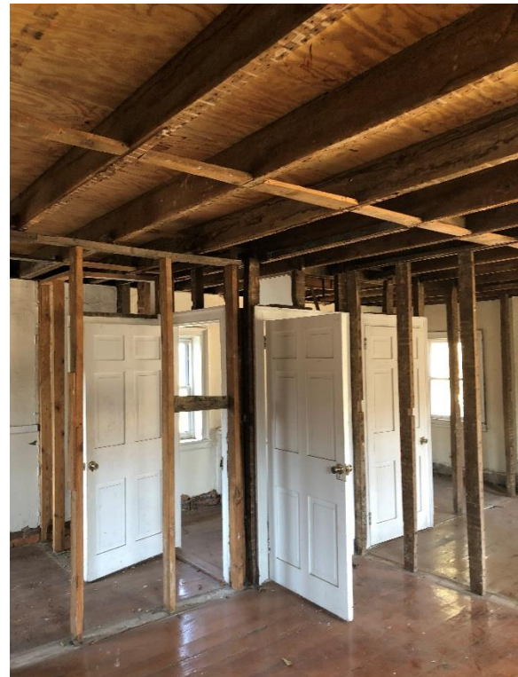
Second floor exposed ceiling/attic floor framing with removed plaster and lath (Mills Group 2018).
