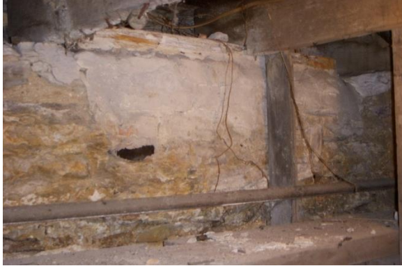
West wall of rear wing cellar showing an area where a window opening in the fieldstone foundation wall has been in-filled (Oehrlein & Associates, 2008)
