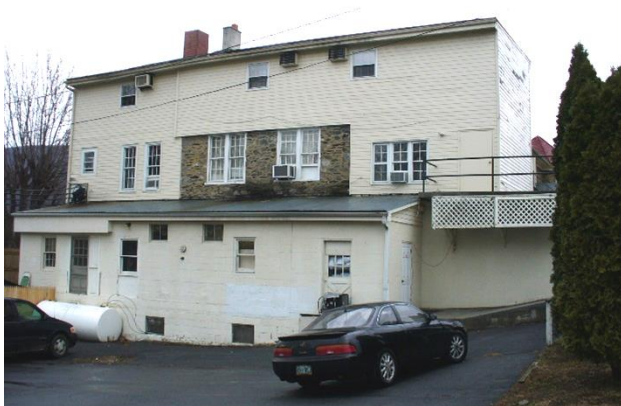
West elevation showing the stone exterior wall of Area 2a. The frame construction at either end (Area 3a and b) and above Area 2a is late 20 th century construction.
