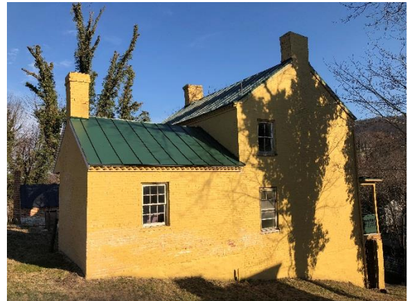
View of new roofing; install new gutters and downspouts for rainwater diversion (Mills Group 2018).
