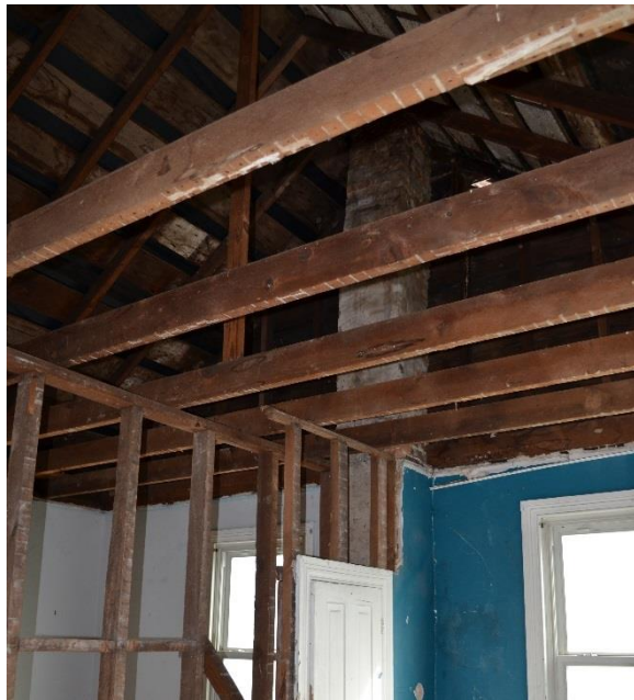
Roof framing over second floor addition to log building, east unit (Mills Group, 2018).
