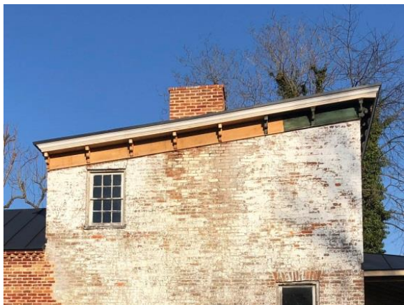
Detail of reconstructed eaves and brackets (Mills Group 2018).
