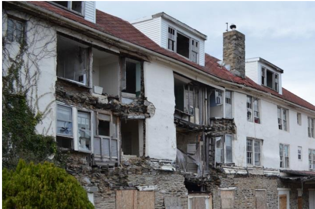
Deterioration along east elevation (Mills Group, 2018).
