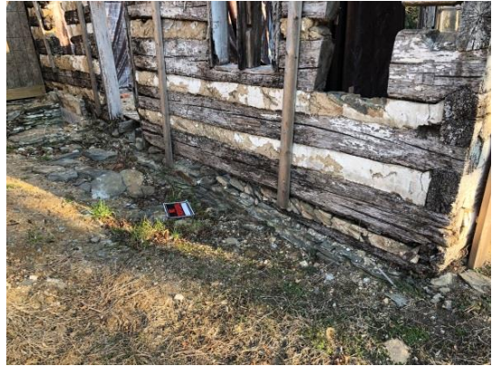
View of deteriorated timber members, West Unit log building (Mills Group, 2018).
