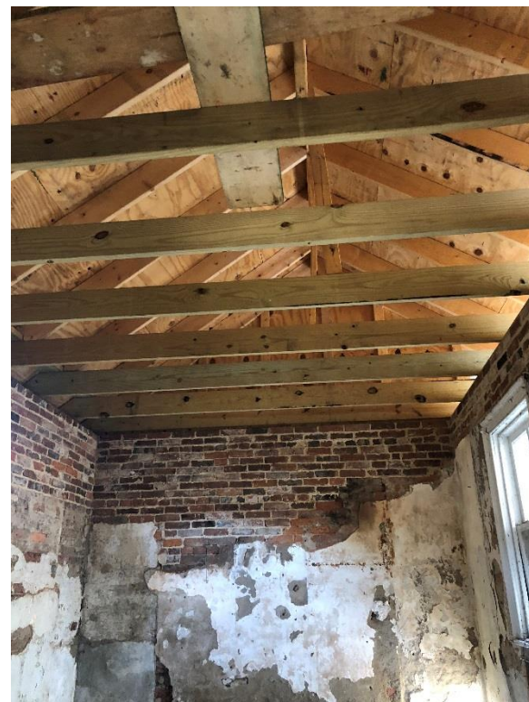
View of replaced roof framing and decking in rear wing (Mills Group 2018).
