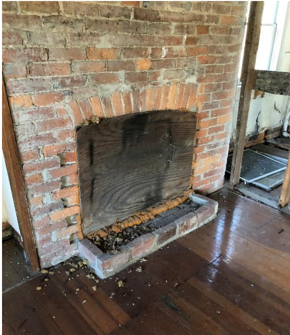
Plywood panel and foam insulation, along with raised brick hearth, at second floor west fireplace (Mills Group 2018).
