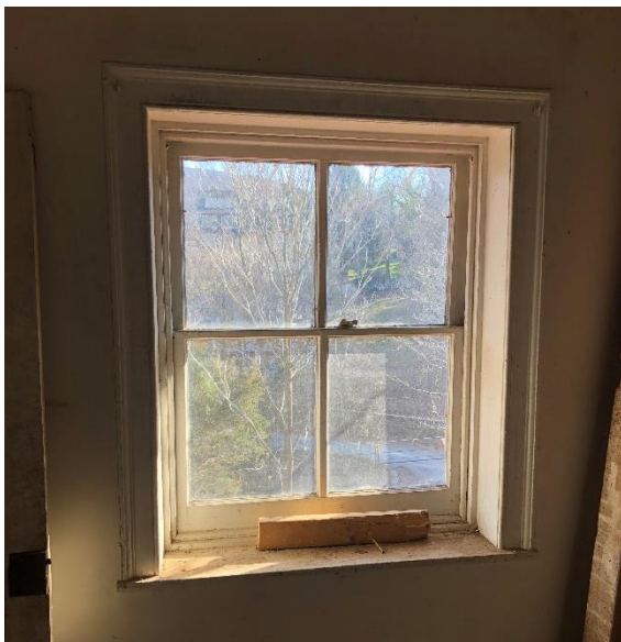
Historic window casing at north window on east wall, second floor (Mills Group 2018).
