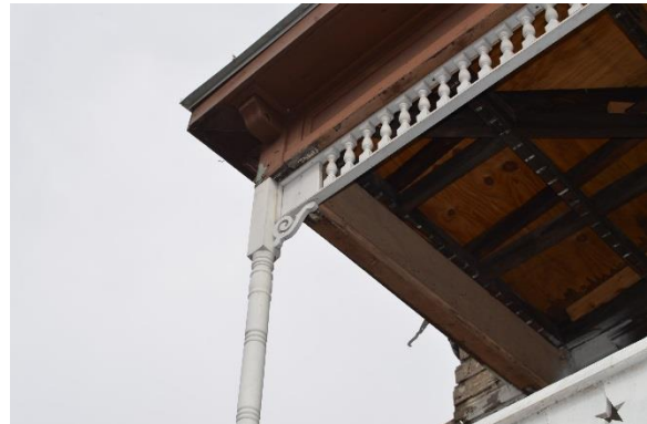
Detail view of west unit porch showing missing ceiling (Mills Group 2018).
