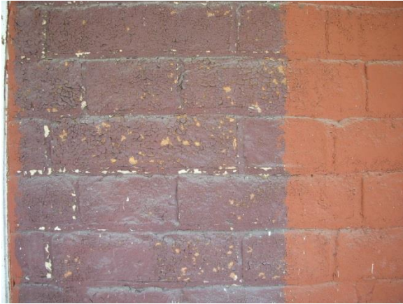
Detailed photograph of painted brick masonry. The red on the right is the most recent color, while the maroon is an earlier paint color. Portions of the original orange brick can be seen in areas of missing paint (Oehrlein & Associates, 2008).
