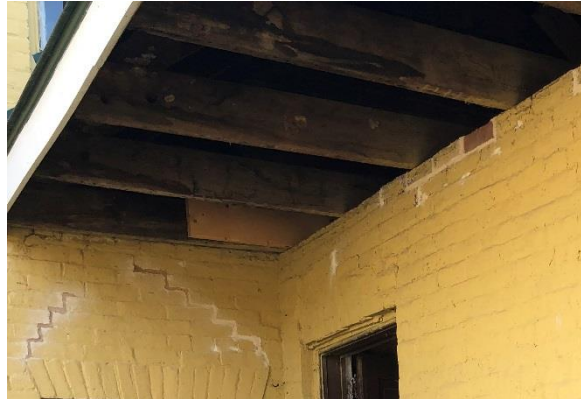
Open rafters on overhanging east side of rear wing roof; replace ceiling/soffit in this area (Mills Group 2018).
