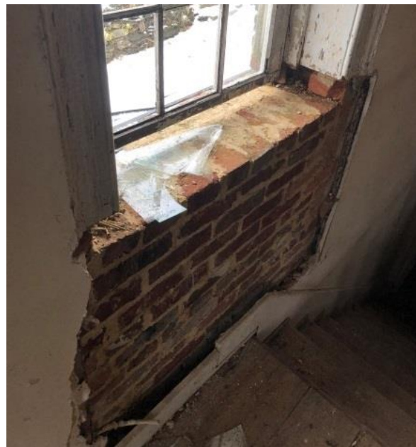
Plaster deterioration under north window, second level (Mills Group 2018).
