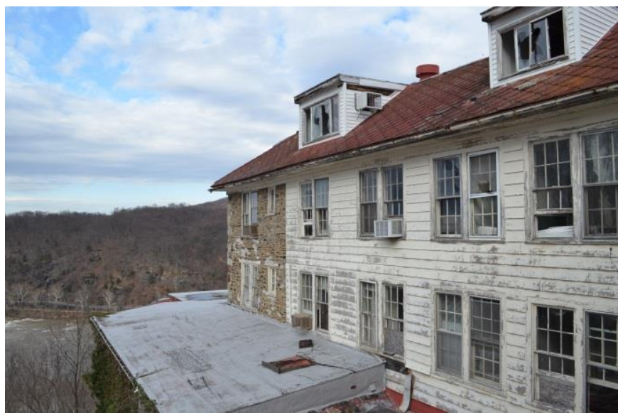
Asbestos shingle roofing (above) and flat seam metal roofing (below) (Mills Group, 2018).
