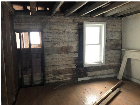
Second floor addition to log building framing visible from first level, east unit (Mills Group, 2018).
