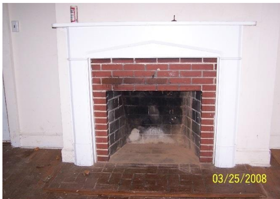
New firebox at east room fireplace, first floor (Oehrlein & Associates, 2008).
