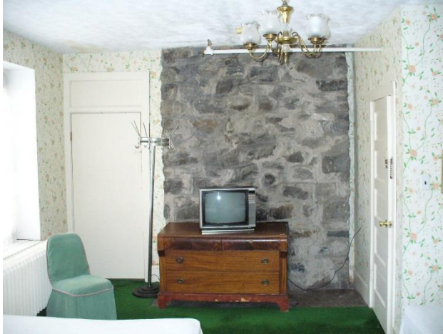
Second floor guest room in Area 2a showing stone fireplace remaining at east wall. The five panel door at the right in the photo may date from the 1920 reconstruction, but all hardware is recent.
