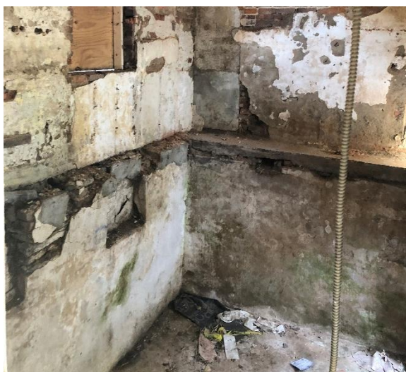
Missing floor framing in rear wing (Mills Group 2018).
