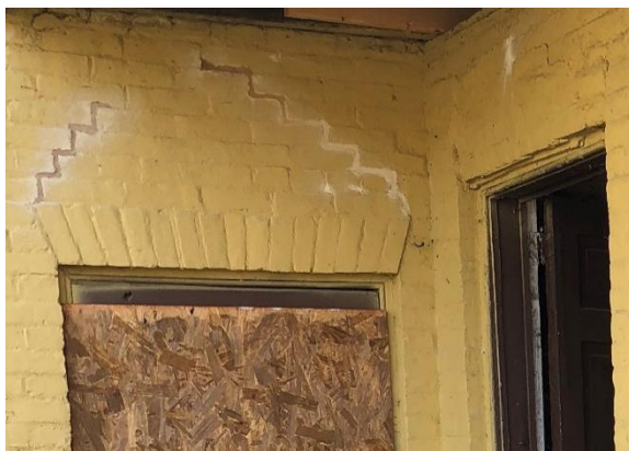
Reconstructed jack arch and adjacent masonry over north exterior door (Mills Group 2018).
