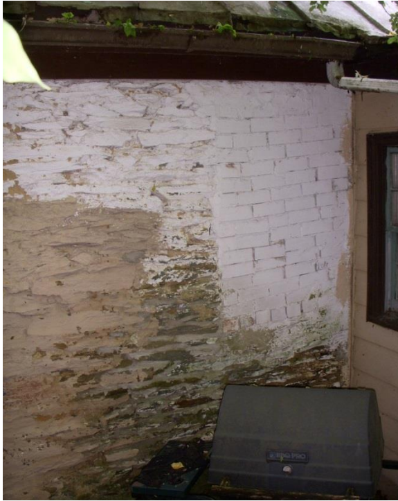
Former window opening in stone wall now filled in with brick masonry (Oehrlein & Associates, 2008).
