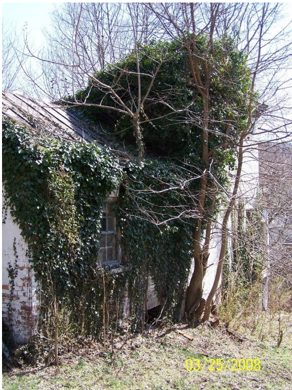
Invasive ivy at west elevation (Oehrlein & Associates, 2008).
