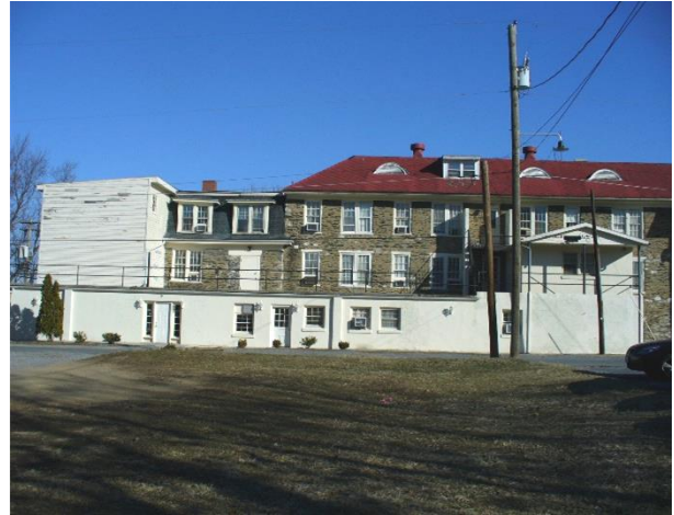
West portion of the south elevation showing the one story Area 9 concrete block construction, the south face of the Area 3b three story frame addition and the Area 3c porch. All are mid to late 20 th century construction.
