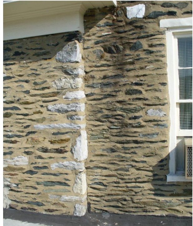
Construction joint between Area 1 (right) and 2 indicates that Area 2 was constructed prior to Area 1. Much of the stonework of Area 1, however, appears to have been more recently rebuilt.
