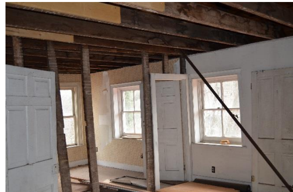
View of interior stud walls with plaster and lath removed; install new interior gypsum board wall finishes and ceilings (Mills Group 2018).
