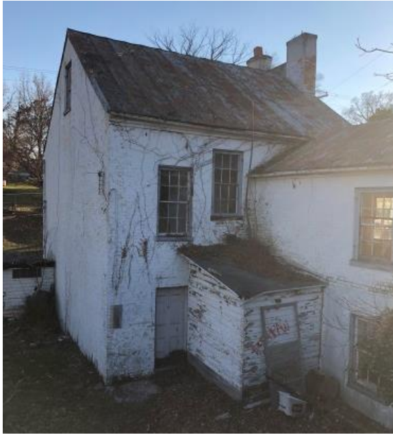
View of deteriorated rear frame addition (Mills Group, 2018).
