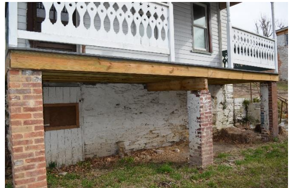
New porch framing, flooring, posts, and balustrade on east unit (Mills Group, 2018).
