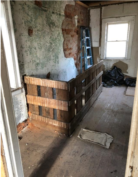
Existing knee wall at north wall of second floor (Mills Group 2018).
