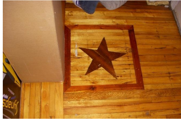
Existing wood flooring at first floor level in east unit log building (Oehrlein & Associates, 2008).
