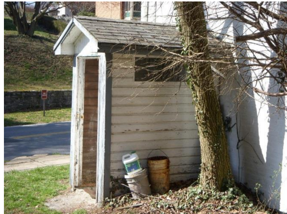
Wood frame stair enclosure addition added between 1922 and 1933 (Oehrlein & Associates, 2008).
