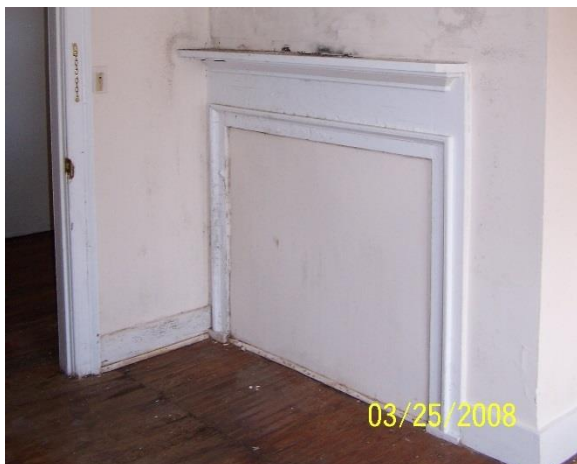
Boarded fireplace in east room, second floor. West room fireplace similar condition. Note brick hearth has been removed at this location and filled with wood flooring (Oehrlein & Associates, 2008).
