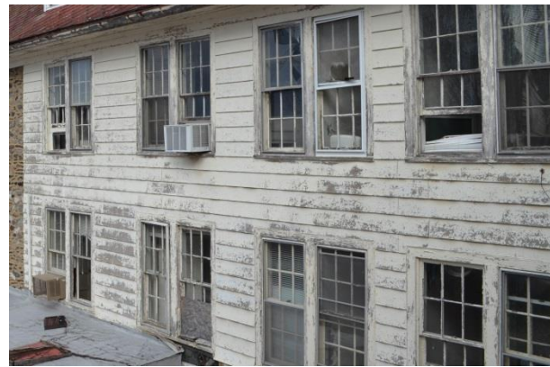
Wood windows and missing windows at stone and frame walls (Mills Group, 2018).
