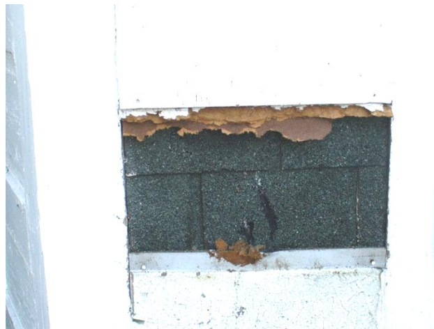
Asphalt shingle siding on the west and north exterior frame wall construction, now covered by pressboard siding.
