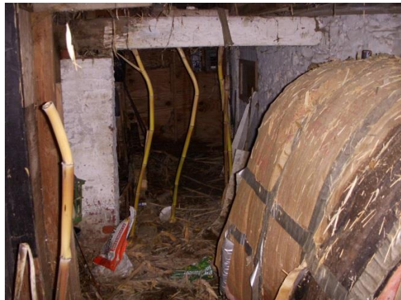
Painted masonry piers under the east unit porch on the south elevation are the only historic element of the porch still remaining (Oehrlein & Associates, 2008).
