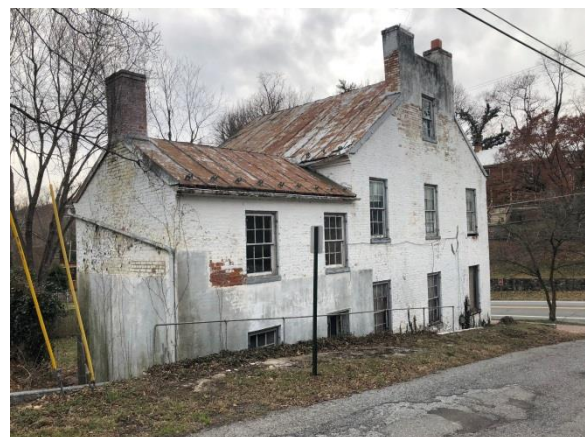
West elevation showing standing-seam metal roof (Mills Group, 2018).
