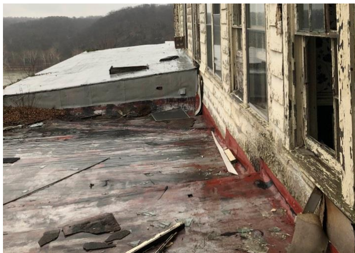
Detail view of deteriorating flat seam metal roofing (Mills Group, 2018).
