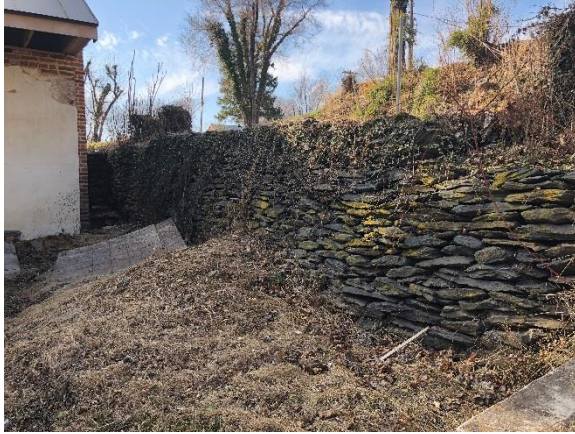
Retaining wall adjacent to rear wing; selectively rebuild with salvaged stone and mortar to match existing (Mills Group 2018).
