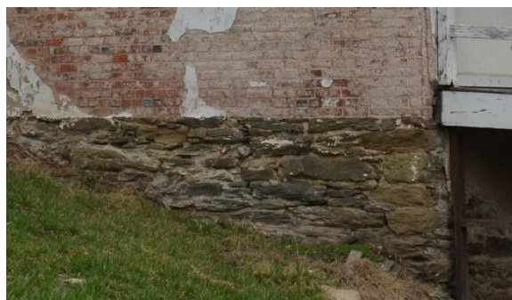
Localized loss of mortar at foundation walls (Mills Group 2018).
