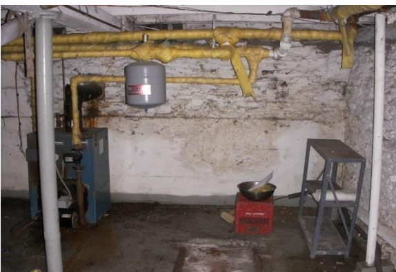
Existing cellar in east unit of log building. The concrete floor slab is not original to the building. All interior walls are whitewashed. Note the supplemental concrete underpinning at the east foundation wall (beyond) (Oehrlein & Associates, 2008).
