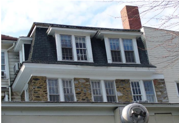
North elevation of Area 2; a two story stone addition with a third story within the mansard roof.
