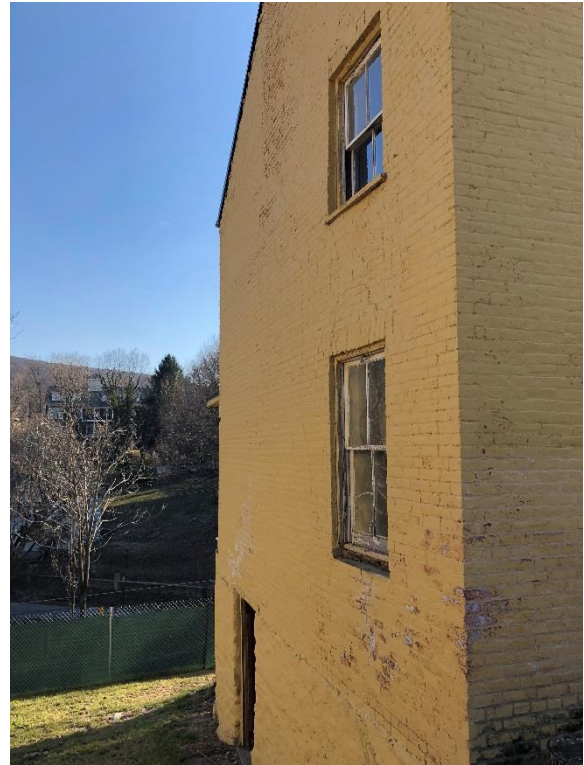
Bulging evident along east wall of main building (Mills Group 2018).
