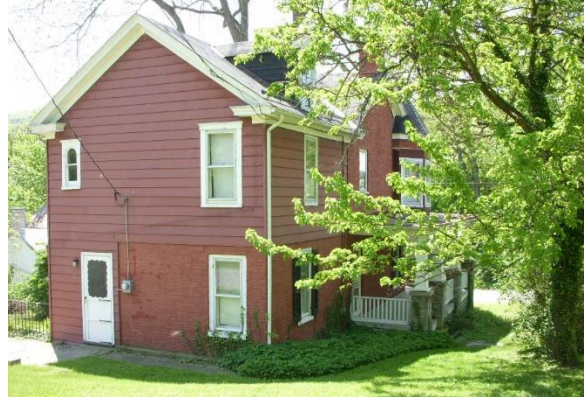
View looking southeast at the rear wing of the house. Note that the original portion of the rear wing is brick, while the later addition is clad in metal siding (Oehrlein & Associates, 2008).
