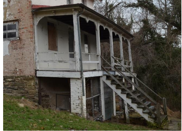
View of south elevation illustrating settlement of masonry porch piers and deterioration of porch framing (Mills Group 2018).
