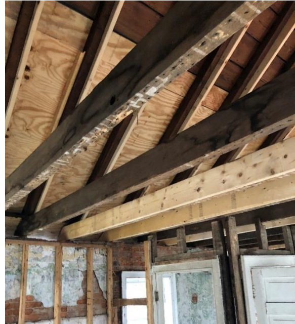
View of north-facing replaced roof decking, sistered rafters, and replaced ceiling joists (Mills Group 2018).
