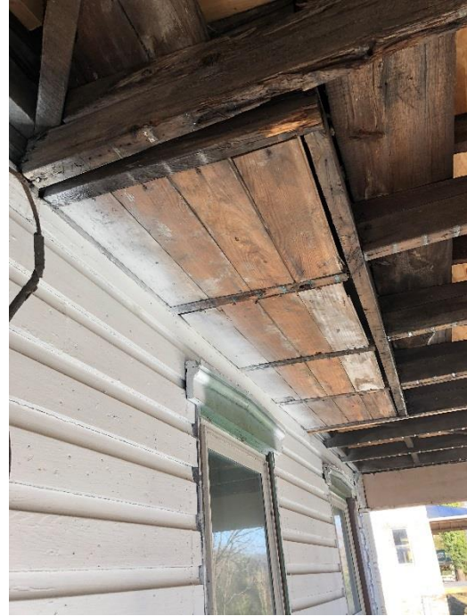
View of floor framing of second level visible from porch (Mills Group 2018).
