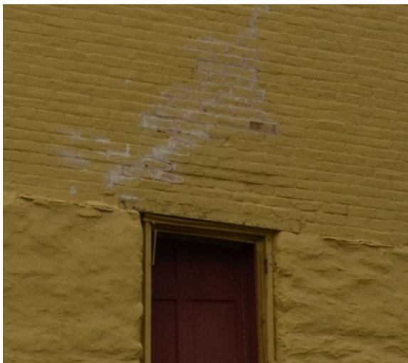
Evidence of bulging and cracking above basement door on east elevation (Mills Group 2018).
