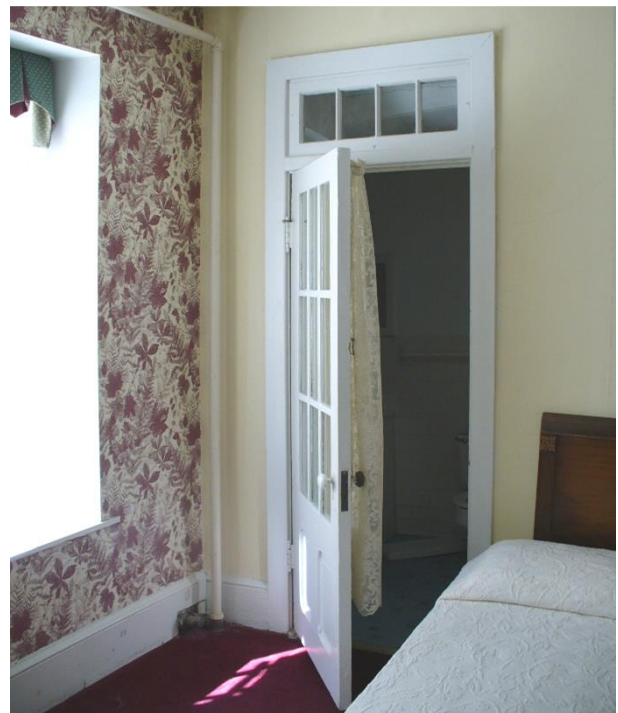
1920's exterior door at the second floor part of the west wall of Area 2 that entered onto the open porch that once existed. The door now provides access to the bathroom located in Area 3b addition.
