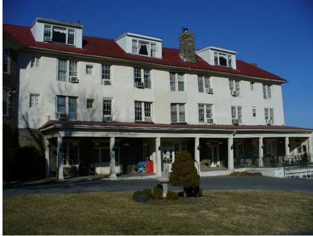
Area 1 south elevation stone wall now covered with stucco. The left portion may be from the 1920 reconstruction or earlier; the right three bays have been recently reconstructed. The frame dormers and the majority of the porch construction are late 20 th century.
