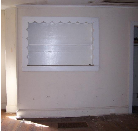
West room fireplace covered with drywall (Oehrlein & Associates, 2008).
