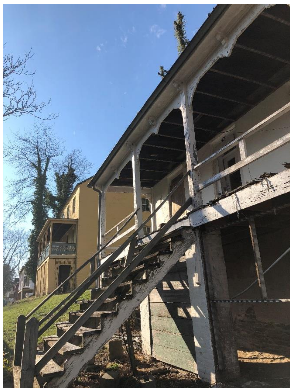
View of missing wood sheathing between masonry porch piers (Mills Group 2018).
