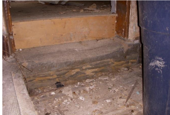
Photograph of modern wood floor framing installed on top of original wood floor in west unit (Oehrlein & Associates, 2008).
