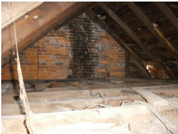
View in attic above rear wing. Note the evidence of a former chimney on the far wall (Oehrlein & Associates, 2008).
