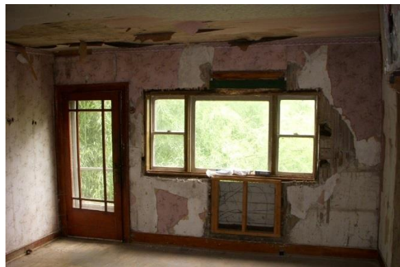
Existing picture window at location of former door opening in west unit (Oehrlein & Associates, 2008).
