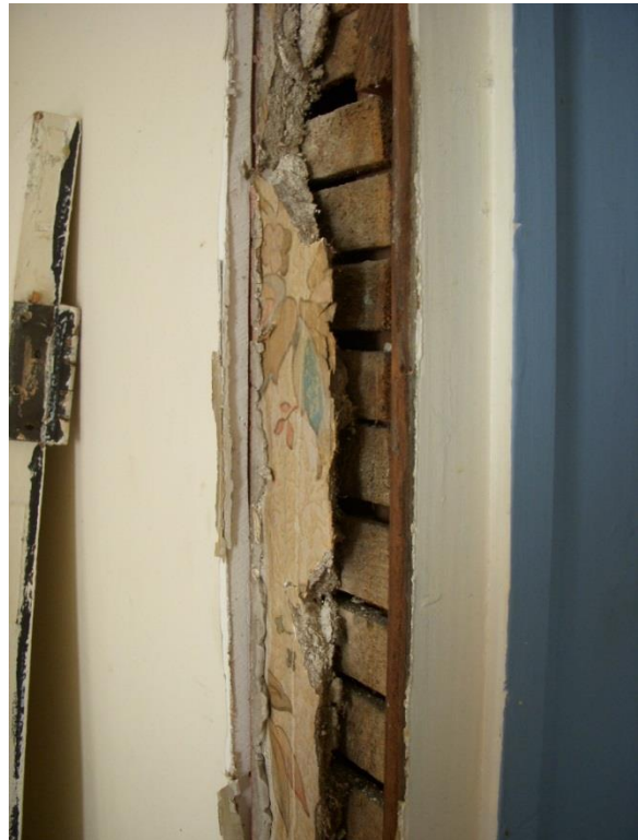
Detailed view of gypsum board installed over historic plaster (and wallpaper) over wood lath (Oehrlein & Associates, 2008).
