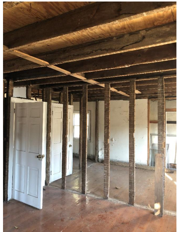
Exposed second floor interior wall framing (Mills Group 2018).
