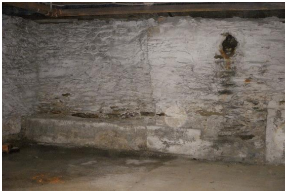
West foundation wall concrete underpinning and concrete ground slab. Note the damp area in the southwest corner where water often collects (Oehrlein & Associates, 2008)
