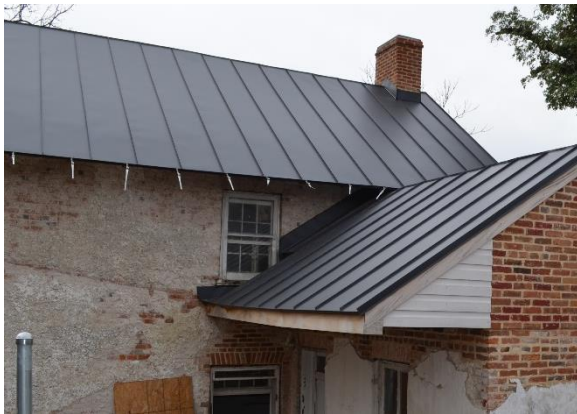
Reconstructed roof form with window cut-out (Mills Group 2018).
