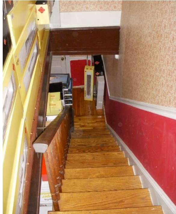
View looking from the second floor down to the first floor in the east unit. Note the missing guardrail on the left side of the photo (Oehrlein & Associates, 2008).
