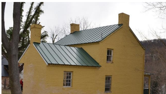
View of new standing-seam metal roof (Mills Group 2018).
