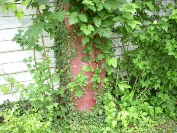
Existing painted CMU chimney on the west elevation of the log building (west unit). This chimney is not original to the building (Oehrlein & Associates, 2008).
