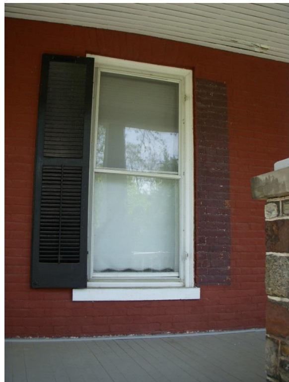
Typical one-over-one wood window with exterior storm panel installed. Only the first floor windows on the south and west elevations under the porch roof have shutters (Oehrlein & Associates, 2008).
