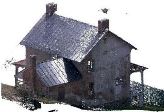
3D Point Cloud scanning of house (Mills Group 2018).
