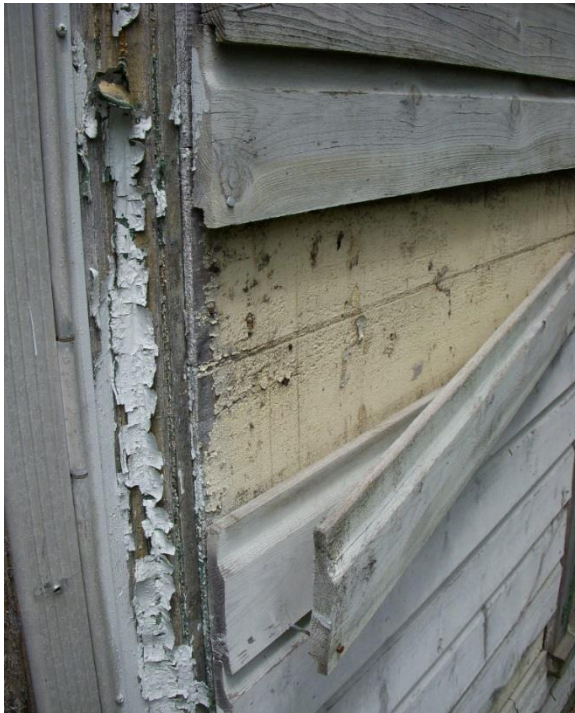
Existing exterior wood siding over older shiplap wood siding on west elevation of west unit log building (Oehrlein & Associates, 2008).
