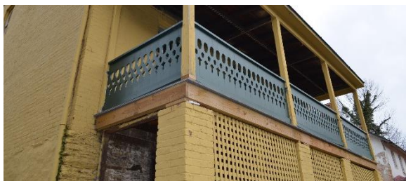
Reconstructed porch railing and rim board (Mills Group 2018).
