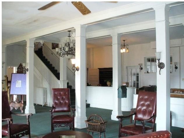
The columns, stair and portion of the reception desk in the lobby appear to date from the 1920 reconstruction of the hotel. The stair to the basement level, office configuration, public restrooms and all finishes and fixtures are much more recent.
