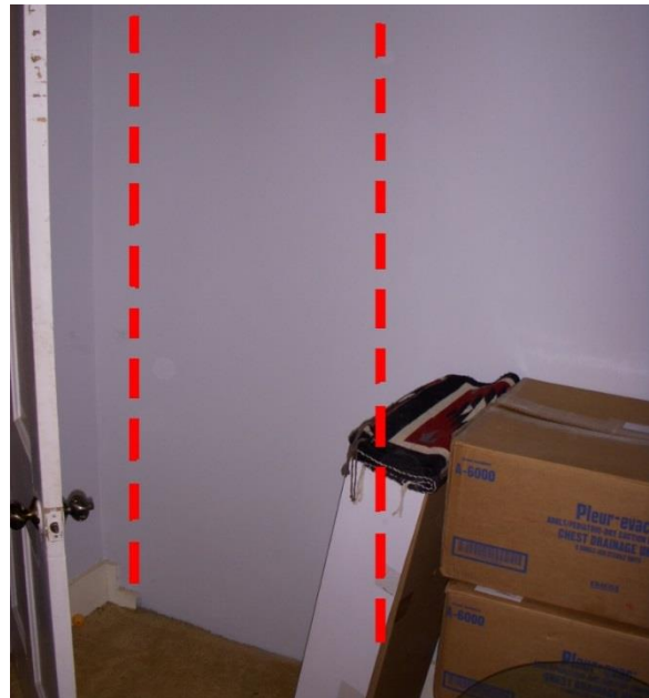
Location of a former door opening at the second floor in the east unit connecting addition to the second floor of the stone building (Oehrlein & Associates, 2008).
