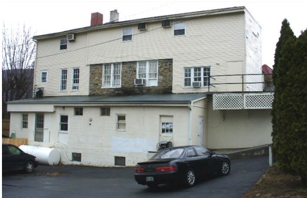
West elevation of the hotel showing the one story Area 8 construction. This recent addition is constructed of concrete block with a corrugated metal roof.
