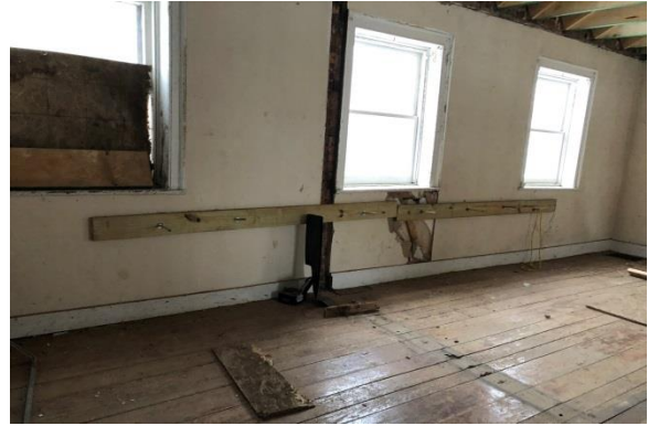
Shoring element on south wall, second level (Mills Group 2018).
