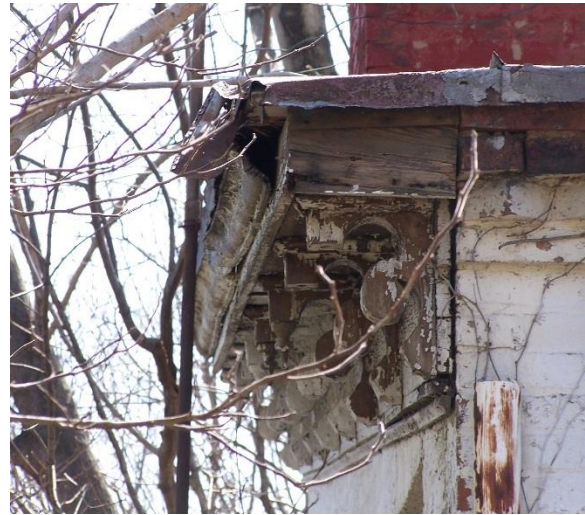
Detail of Italianate wood cornice and brackets at shed roof of main building (Oehrlein & Associates, 2008).
