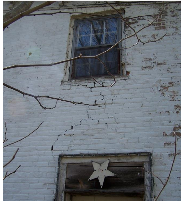
Masonry opening added at east elevation. Note crack in mortar joints above door (Oehrlein & Associates, 2008).
