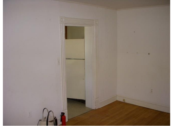
Door opening in original east exterior masonry wall of rear wing that now leads to the addition added on the east side of the rear wing (Oehrlein & Associates, 2008).
