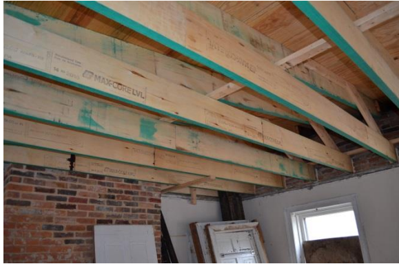
Reconstructed roof framing (Mills Group 2018).
