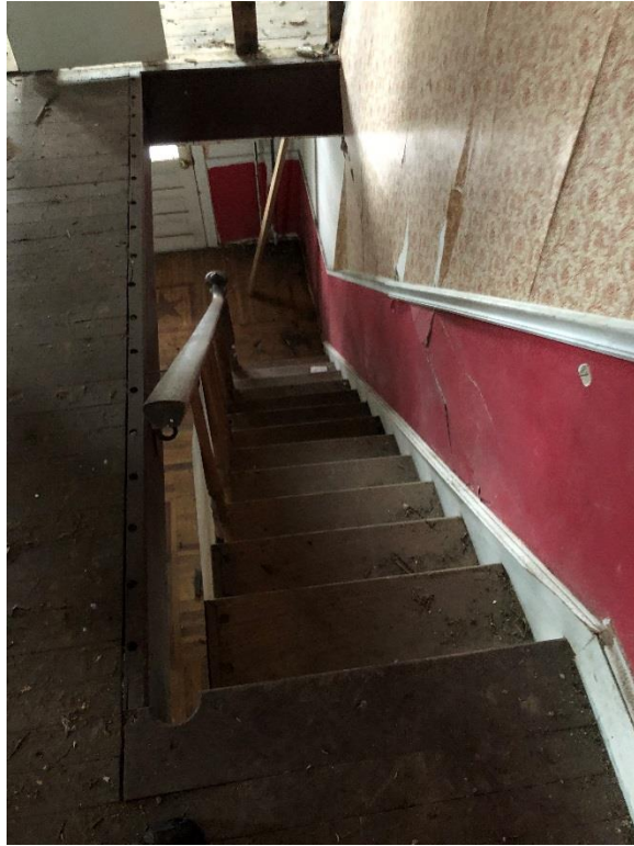
View of settlement of East Unit stairs from level 1 to level 2 (Mills Group 2018).
